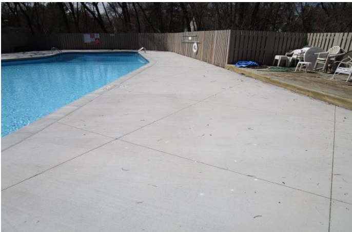
New north pool deck
