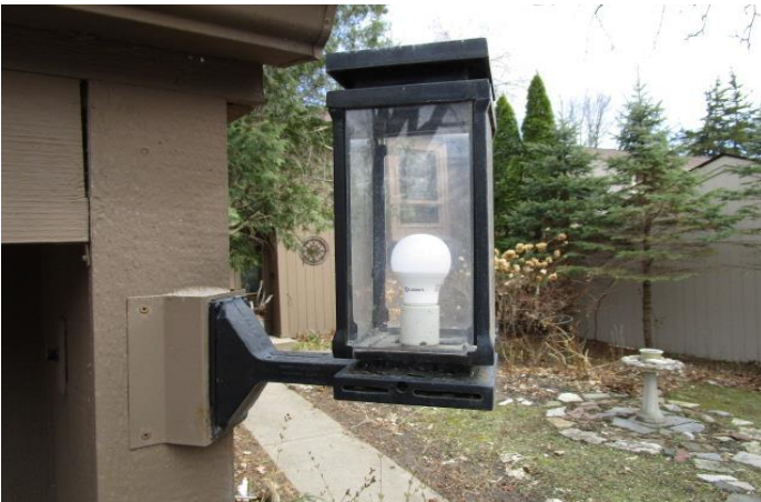
Light fixture at single family home garage
