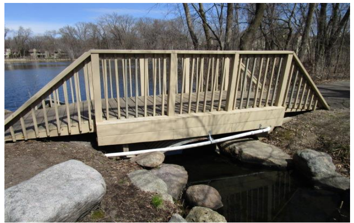
Bridge with railings
