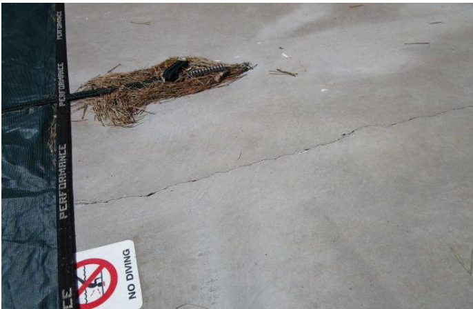
South pool deck in good condition
