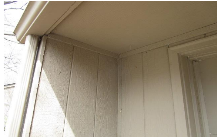
Soffit, siding and trim
