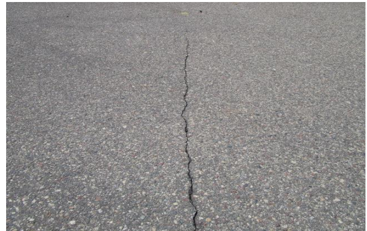
Transverse crack
