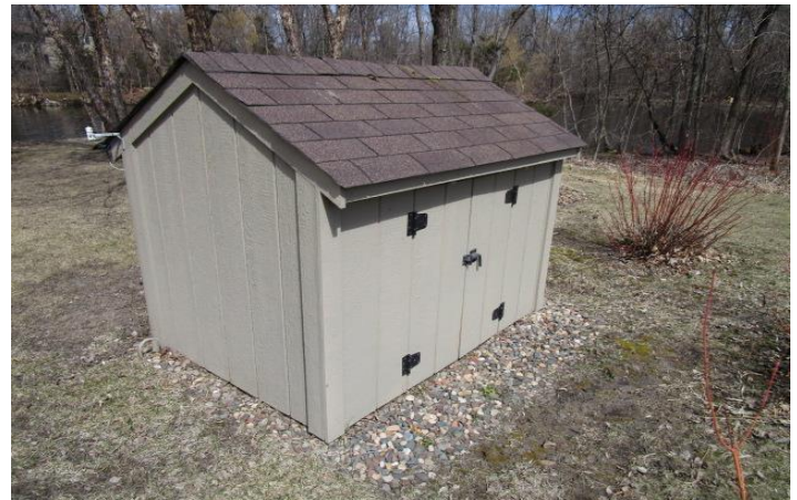
Shelter for irrigation equipment
