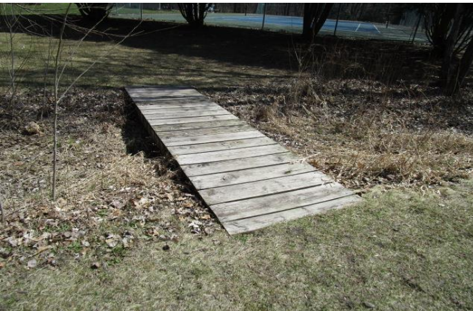
Bridge without railings
