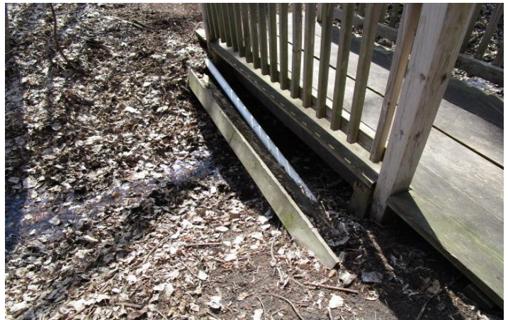
Beam under bridge
