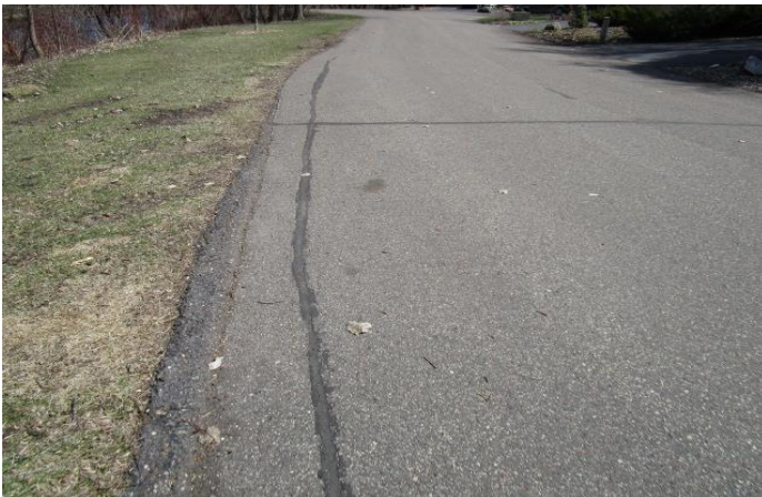
Previous crack repair
