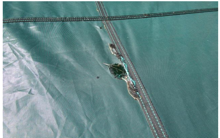
Tear at south pool cover
