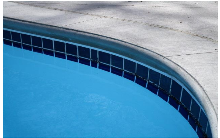
Concrete coping and waterline tile
