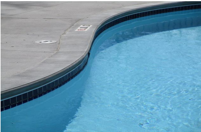
Concrete coping and waterline tile
