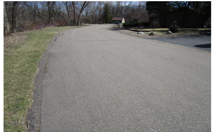
Street pavement in good condition
