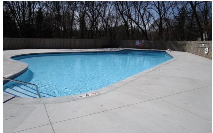
New north pool deck
