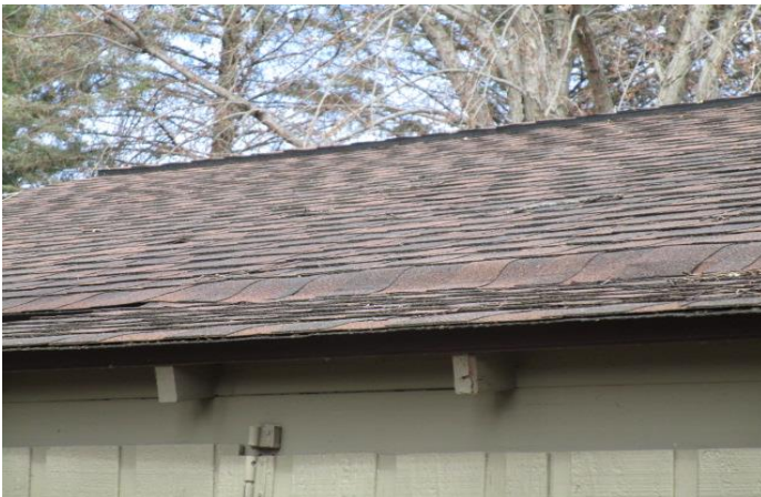
Shingles at roof
