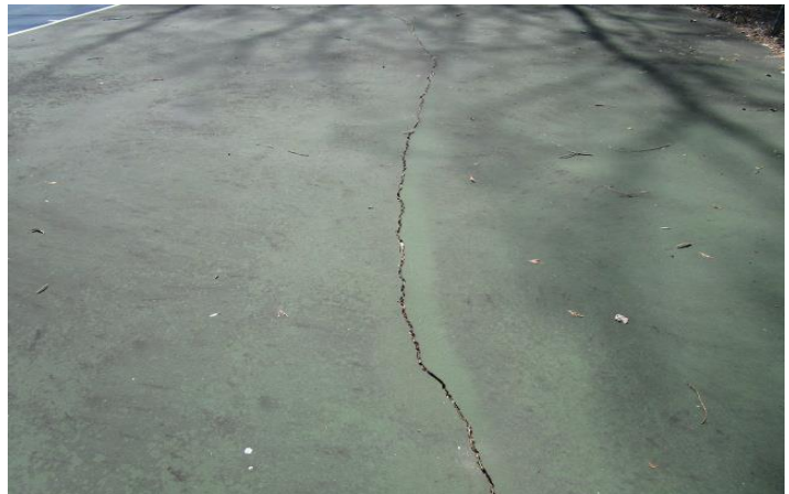
Pavement crack
