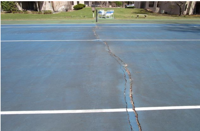
Pavement crack
