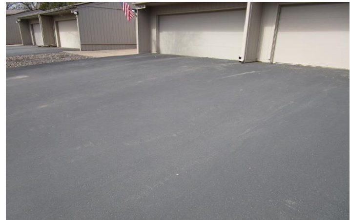
Driveway seal coat in good condition
